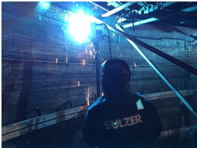
Picture 1: On site coker drum repair
