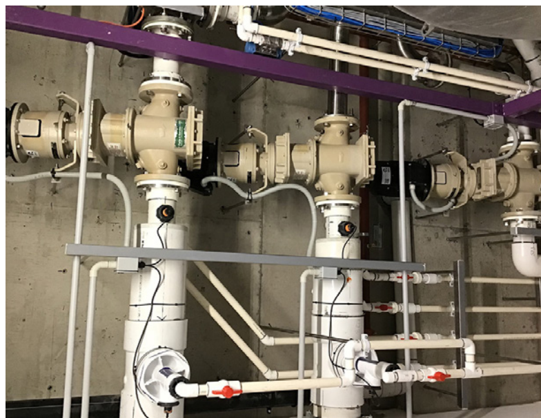
Sulzer supplied three of its 10K Series Muffin Monster Grinders, built to the hospital's specification.
