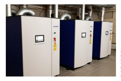
Single stage kinetic blowers with high speed motor drive and magnetic bearings, such as the HST™ turbocompressor by Sulzer shown here, have become the preferred choice for waste water treatment applications in recent years.
